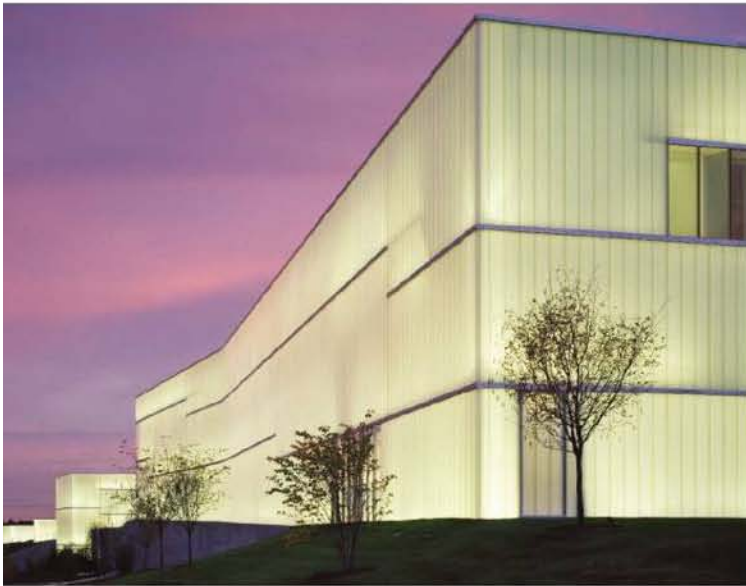
The Nelson-Atkins Museum of Art Bloch Building features five 'lenses' of custom glass channels in a double-glazed curtain wall application.
