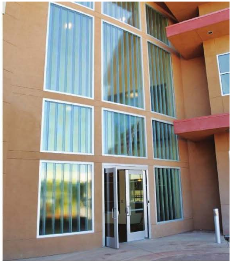
The Ceres Community Center (California) uses channel glass as an aesthetic feature for the building.
