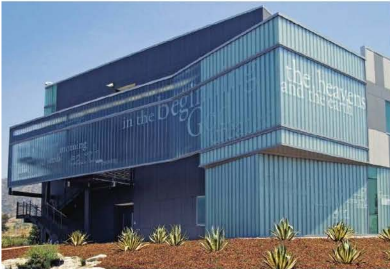
At Azusa Pacific University's (APU's) Segerstrom Science Center (Azusa, California) the single- and double-glazed walls of obscuring channel glass combine privacy with light-scattering properties.
