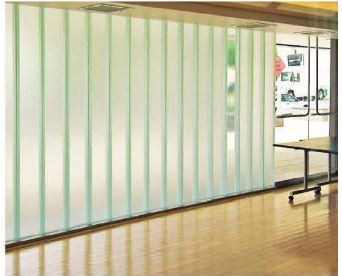
Westwood Branch Library (Los Angeles, California) uses channel glass walls and partitions to admit and distribute large amounts of natural light into the building.
