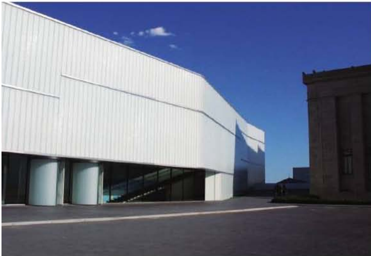
Vertical channel glass systems allow for virtually unlimited glass façades without interim frame support.
