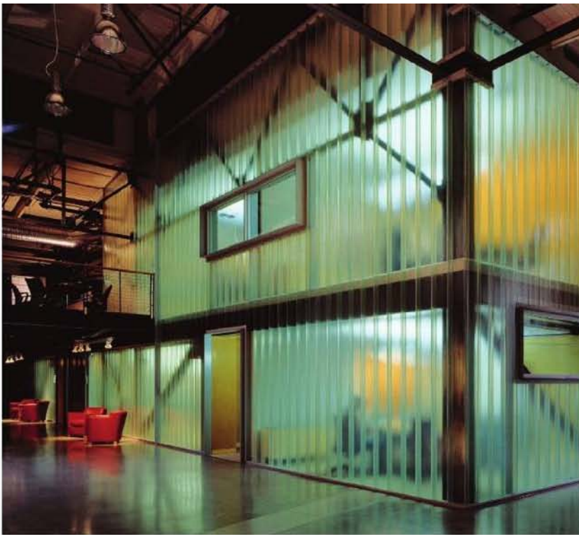
Channel glass is a translucent, roll-formed, U-shaped cast glass that can create sweeping walls of glass of unlimited width without vertical aluminum framing. Note the all-glass corner at the San Francisco, California, building.
