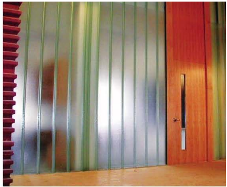
For either exterior or interior applications, various framing systems are available for both single- and double-glazed and vertical or horizontal configurations, as shown here at the Genomic Center (Princeton, New Jersey).
