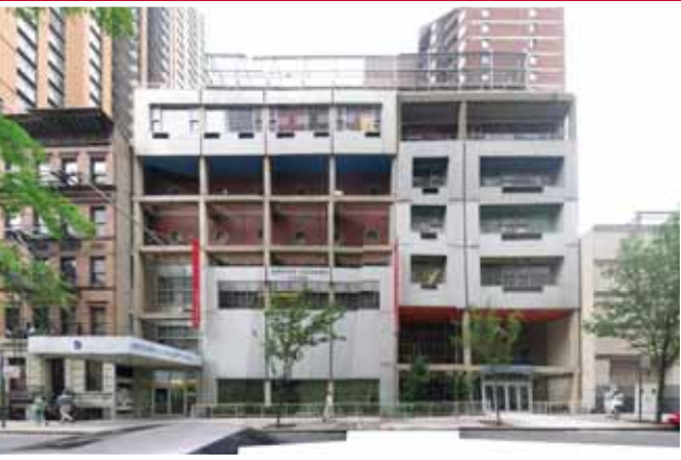
The building before renovation.
