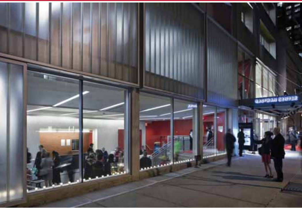
The addition of translucent channel glass makes for a more attractive exterior.
