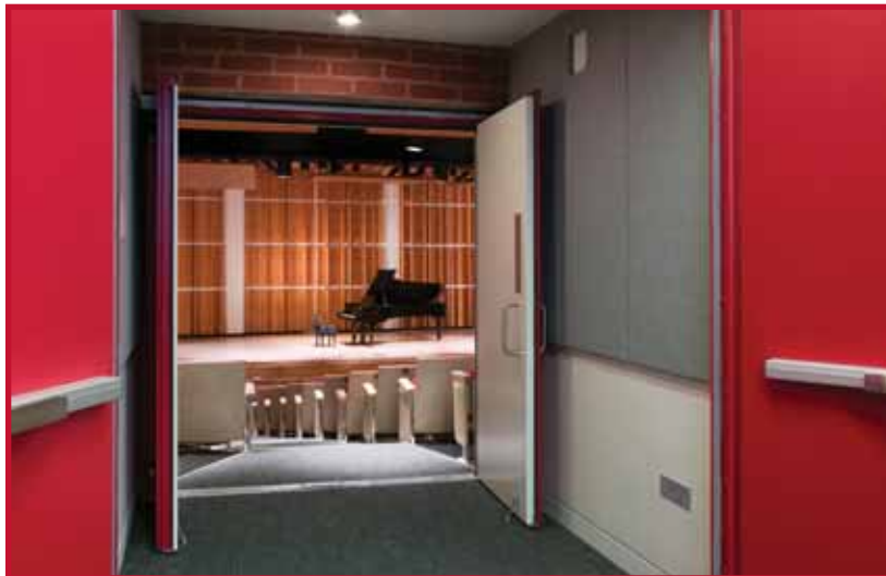
The addition of sound locks provides acoustical isolation.
