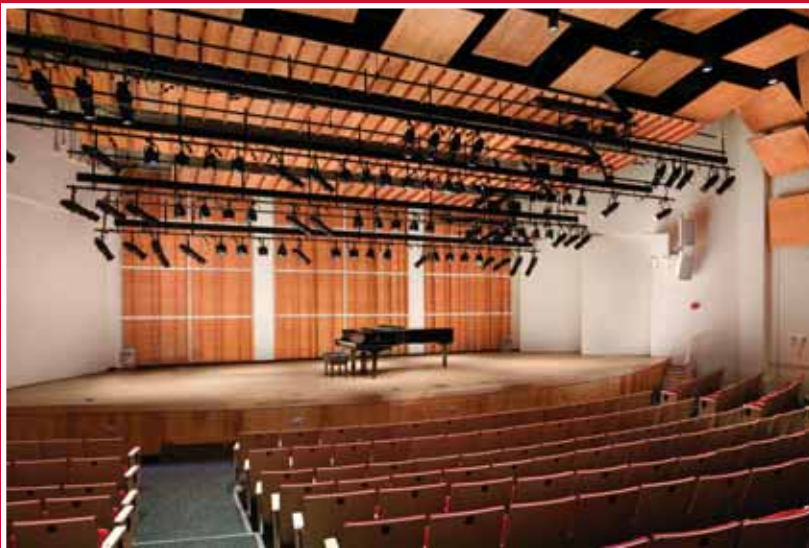
Top and bottom: Two views of the motorized rigging system from JR Clancy.
