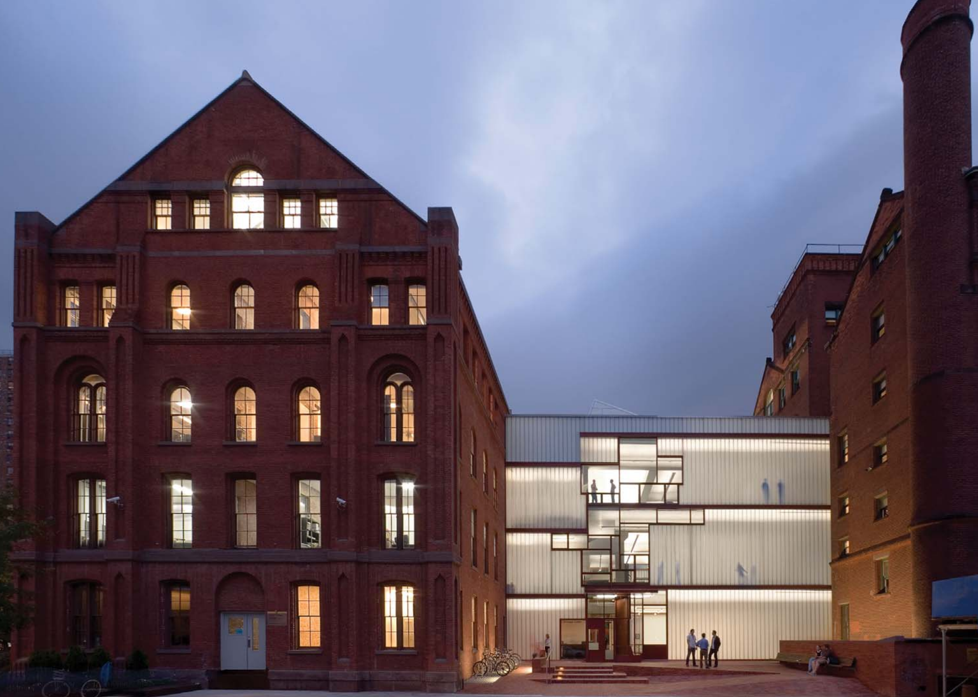
2005 Pratt Institute School of Architecture, Higgins Hall. From left to right: North Wing, Central Wing, South Wing
