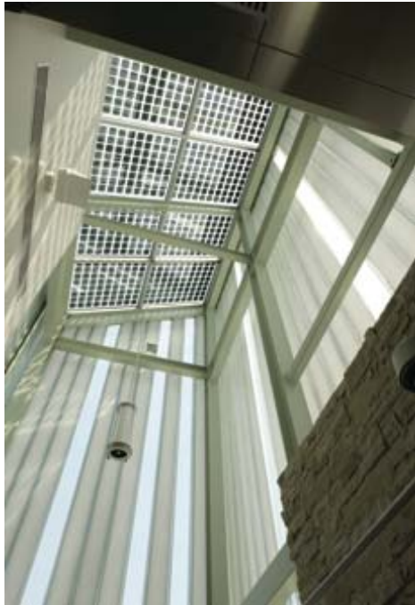
THERE IS LOTS OF THOUGHTFUL DETAILING, SUCH AS THE CLEAR CHANNEL GLASS AND PHOTO VOLTAIC ROOF, BOTH OF WHICH CAST INTERESTING SHADOWS IN THE SPACE IN ADDITION TO SERVING A FUNCTIONAL PURPOSE.
